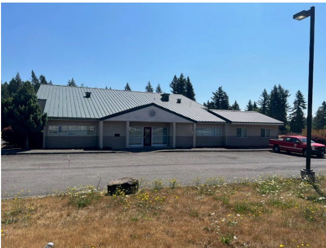
Station 93-Partially Leased to Department of Natural Resources(DNR) and Reserve Apparatus 121 NE 312th Avenue, Washougal, WA 98671
