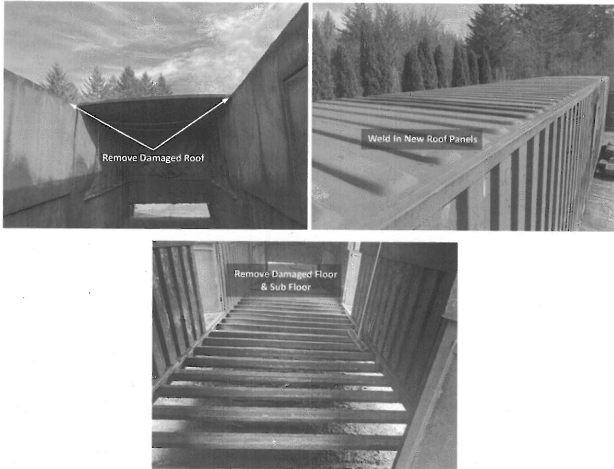
Figure 6. Work Completed to Date
